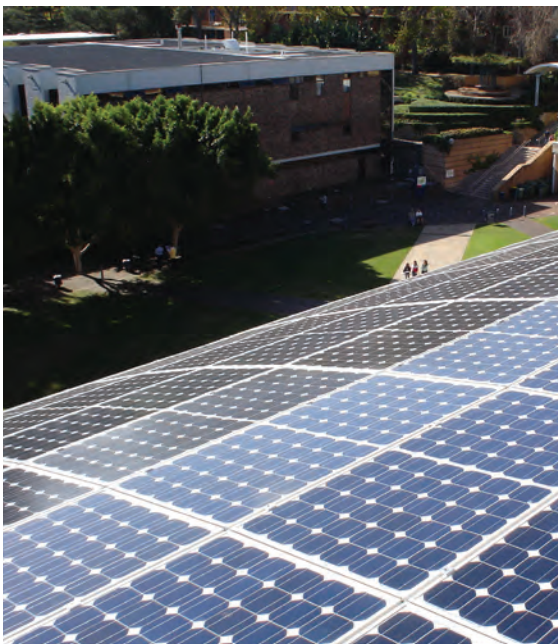
Fig 27. On-campus power generation, Roof - Quadrangle building
